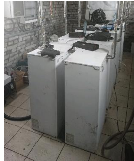
Heat Batteries installation at a trial site (Katowice)
