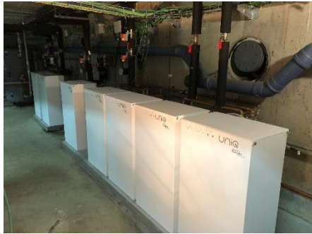
Heat Batteries installation at Kubik
