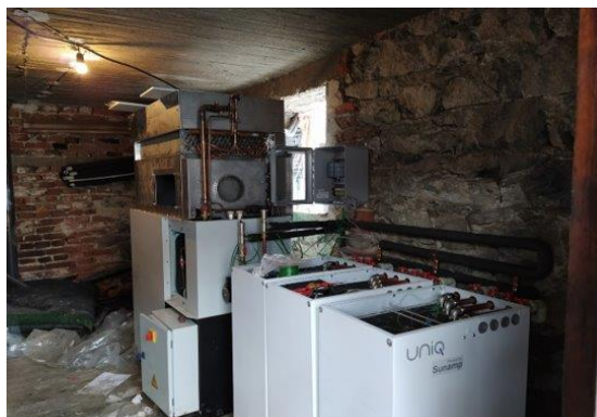
Figure 11 Heat Batteries
